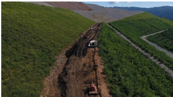
Image 5. The use of FABA as Roadbase material [7]
