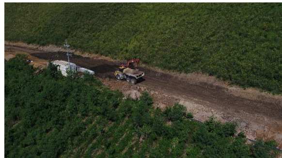
Image 5. The use of FABA as Roadbase material [7]
